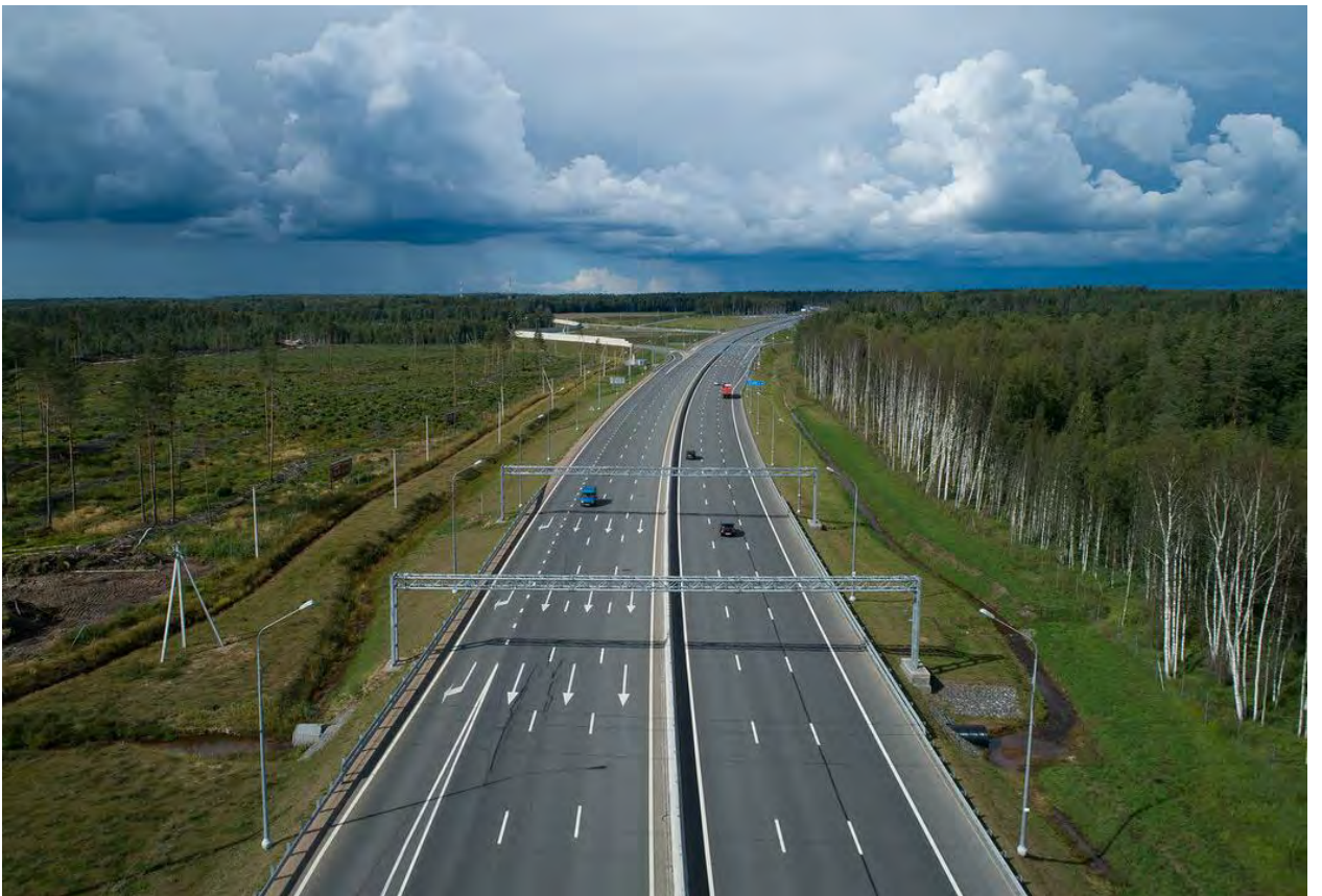
Picture 6. Reconstructed section of the "Scandinavia" highway (part 4)
