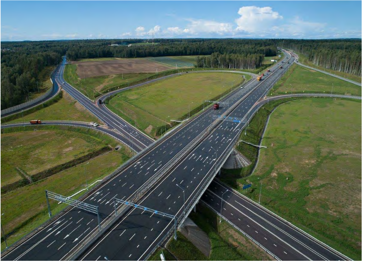
Picture 5. Reconstructed section of the "Scandinavia" highway (part 3)
