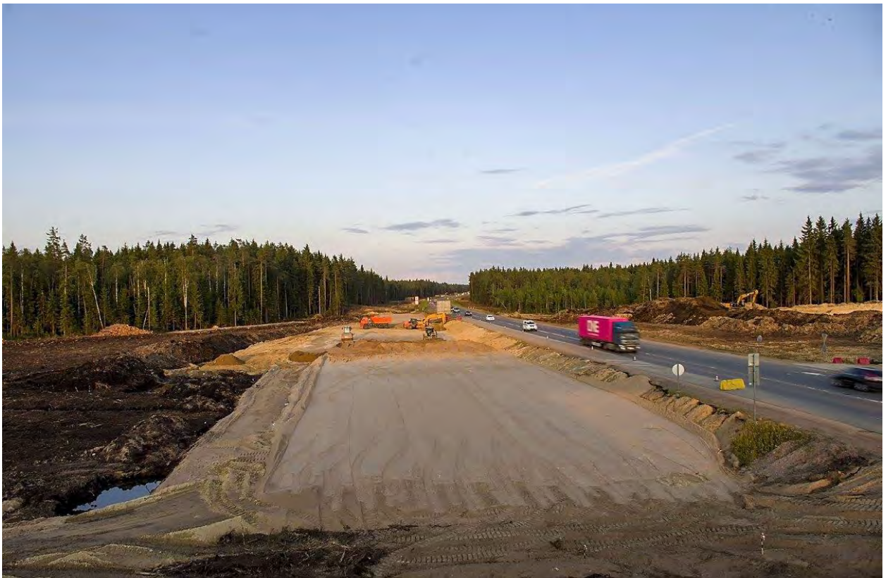
Picture 4. Reconstructed section of the "Scandinavia" highway (part 2)
