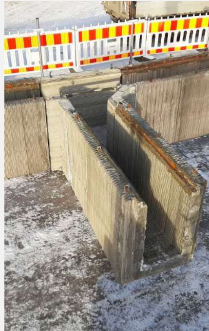
Trenches and Nodes
