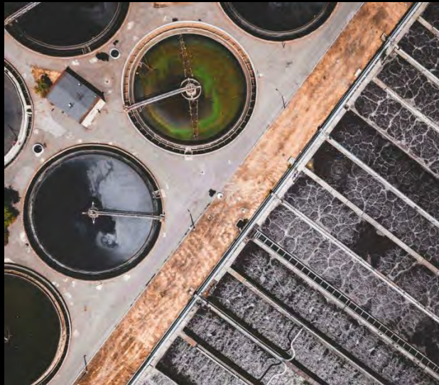
Wastewater treatment facilities
